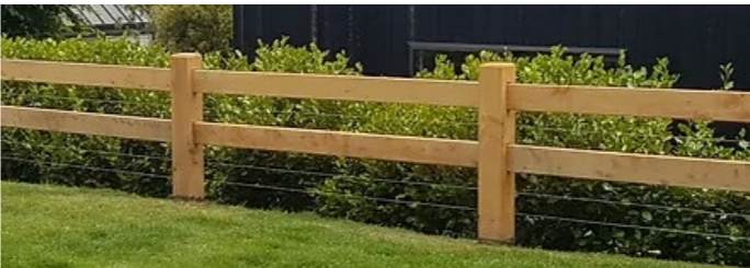
Figure 11. Post and rail fence
