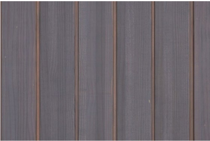
Timber cladding may be weatherboards, including the use of shiplap and tongue and groove profiles in either vertical or horizontal orientations.
